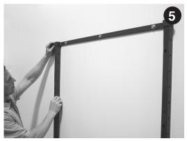
Insert side rails. Do not tighten bolts yet.
