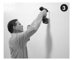
Using a 9/32" bit, drill pilot holes for top crossbar. For masonry walls, pre-drill using 1/4" masonry bit followed by 5/8" masonry bit. Insert lead anchor.
