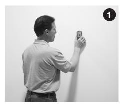
Locate 16" studs on center. All crossbar holes must hit studs in wall. This step not required on masonry walls.
