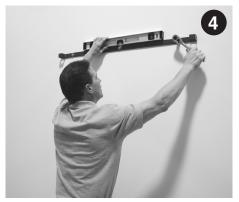
Tighten lag bolts with 9/16" socket wrench. Confirm leveling before final tightening.
