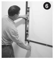
Bolt lower crossbar to side rails. Plumb side rails, mark holes. Pre-drill using 9/32" bit. Tighten lower crossbar bolts.
